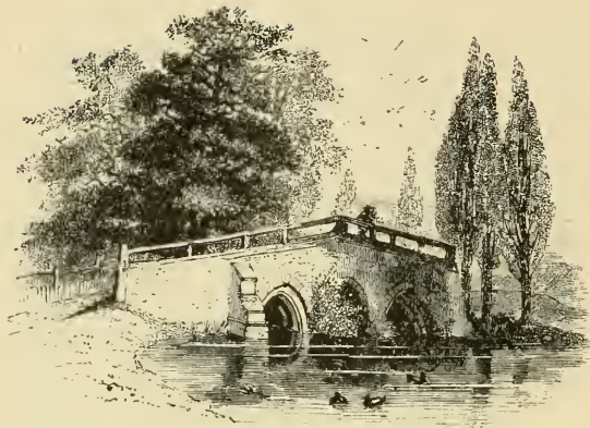
BRIDGE AT HADLEIGH.
